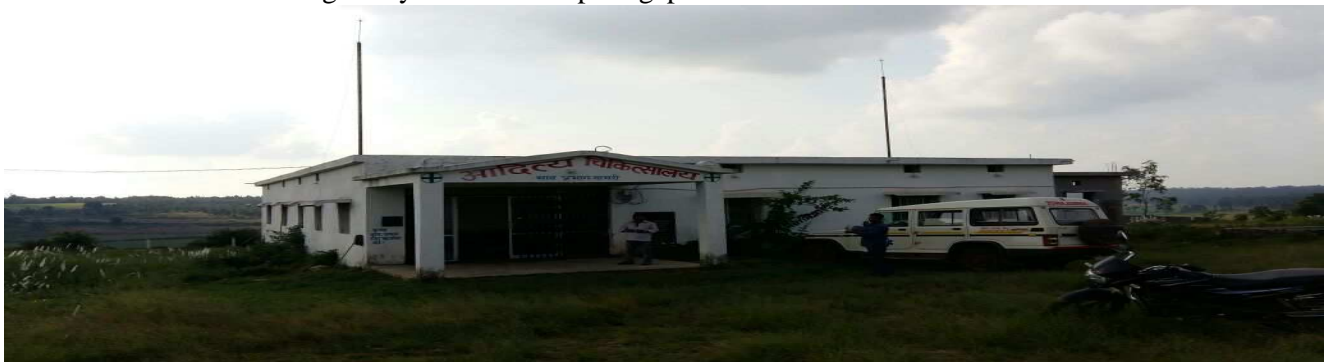
(Lightening Arrester Set At Aditya Chikitsalay Kusmi)
